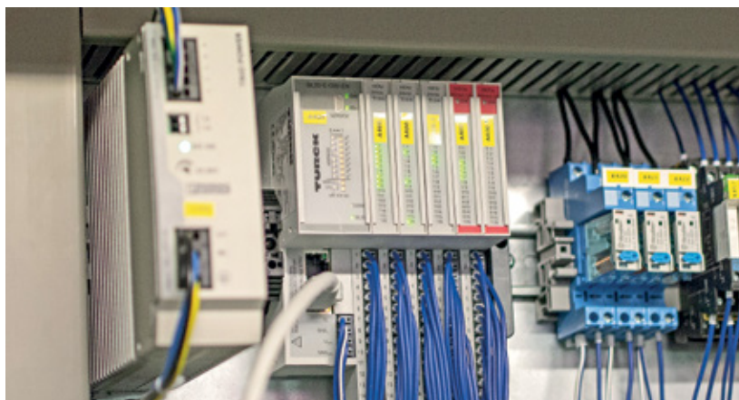
Turck's BL20 I/O system takes care of the signal processing in the control cabinet
